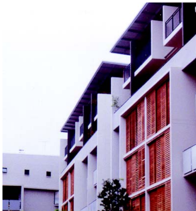
Figure 6.2.3 Use of sun and privacy screens, balconies, roof overhangs and colour give the building individuality.
